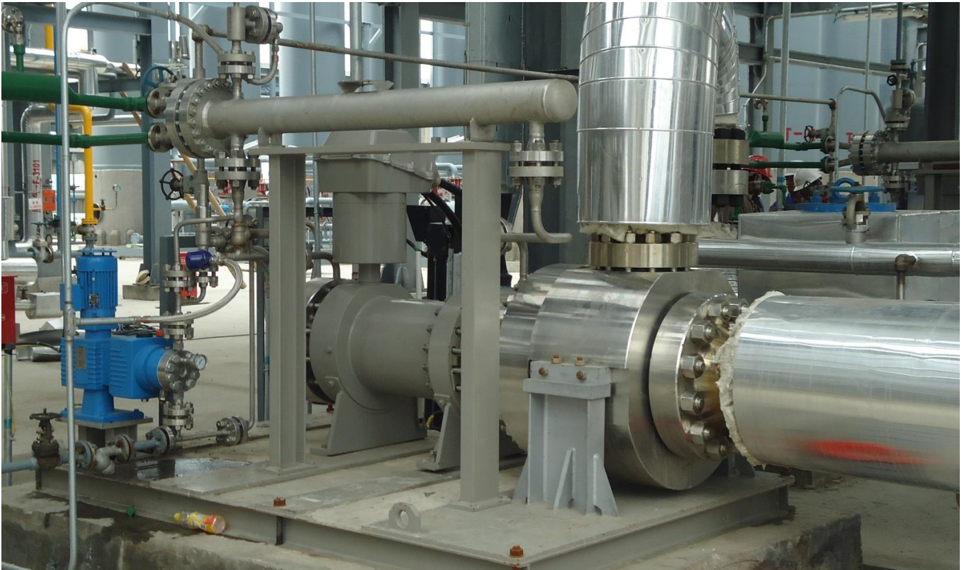
High temperature canned motor pump (image courtesy of Hermetic Pumpen)
